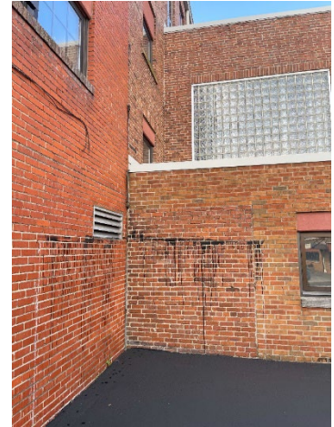
Exterior Walls of Building
