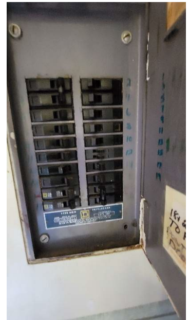
Typical Panel in Original Construction
