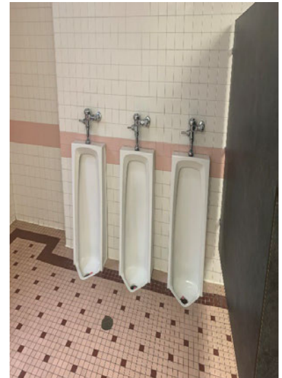
Floor-Mounted Urinals with Manual Flush Valves
