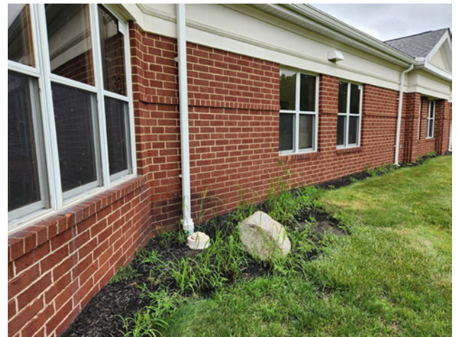
Exterior walls and downspout
