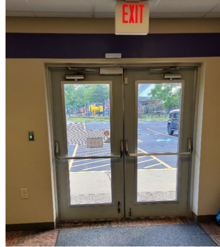
Exit Sign in 1970 Addition
