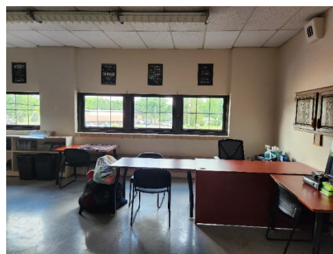
Second Floor Windows
