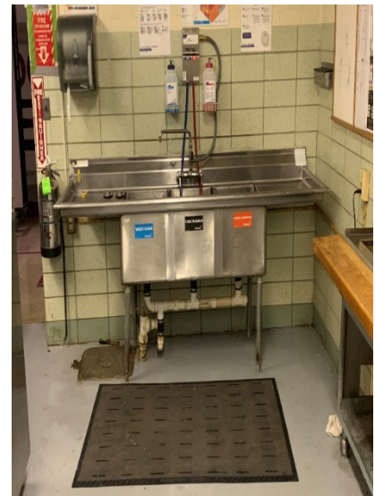
(3) Compartment Sink w/Grease Trap
