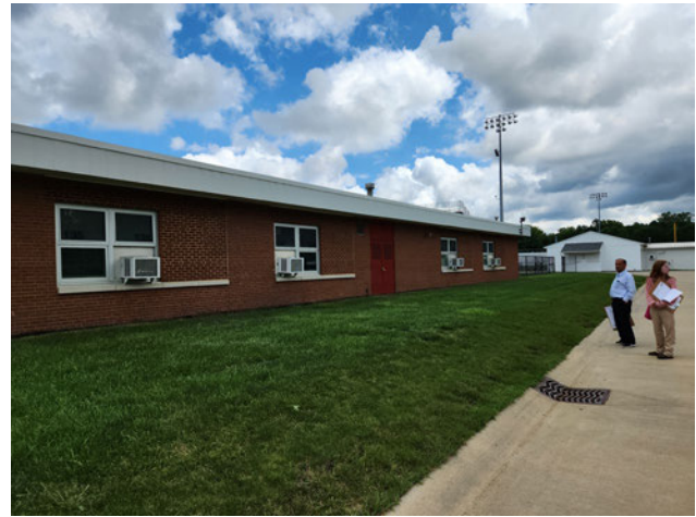
Exterior Brick and Control Joints
